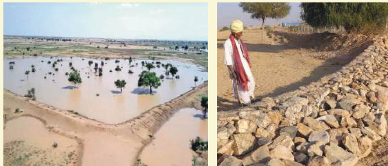
Fig 7-8: Khadeens in Rajasthan, are created on slopes of farm lands by building a 'bund' that catches surface run-off after it rains.
